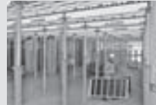
Slab Formwork
