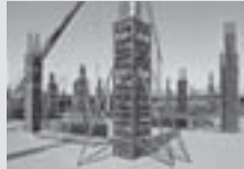
Column Formwork
