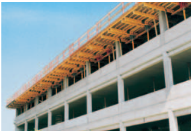
Cantilevered PERI UNIportal edge tables with guardrails.
