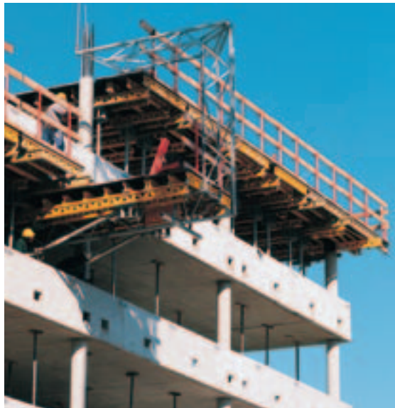
Vertical moving of PERI slab tables.
