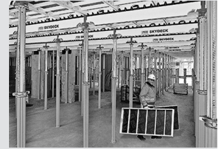
Slab Formwork
