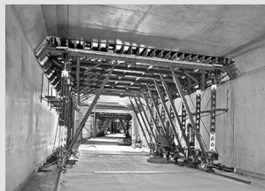
Tunnel Formwork
