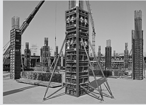
Column Formwork
