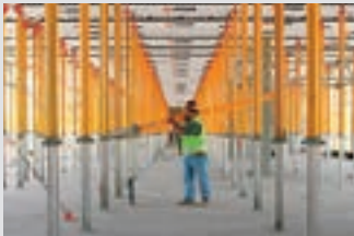
Slab Formwork
