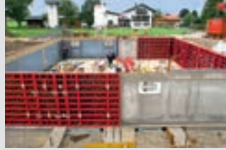
Wall Formwork
