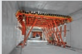
Tunnel Formwork
