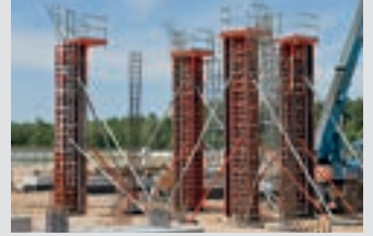
Column Formwork
