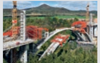
Bridge Formwork
