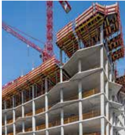
Slab tables with GT 24 Girders and steel walers can be planned and assembled according to specific geometries. The units can be quickly moved with the help of a transportation fork.
