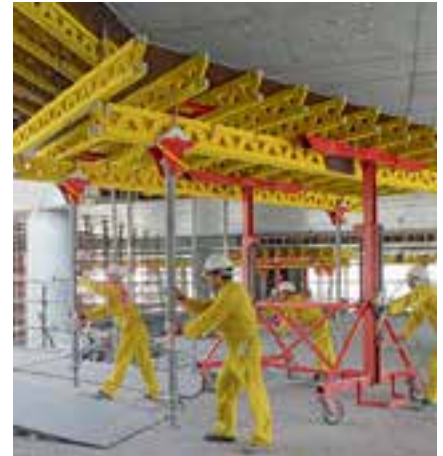
In particular, for large slab thicknesses and high loads, slab tables are configured with the high load-bearing GT 24 Formwork Girders.
