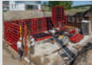
Wall Formwork
