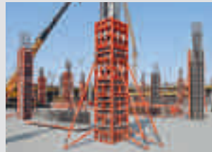
Column Formwork
