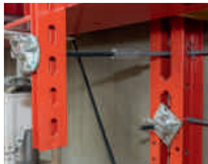
Horizontal loads at right-angles to the level of the main beam frame are transferred directly from the Main Beam HDT into existing structures e.g. abutment.
