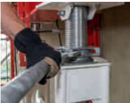
The Wing Nut Spanner HD is used to release the Compression Brace Spindle HD, Head Spindle HDK 45 or spindles fitted with the Adjusting Nut TR 110.
