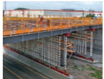
HD 200 as main beam section for the building of a road crossing using a steel composite construction method.
