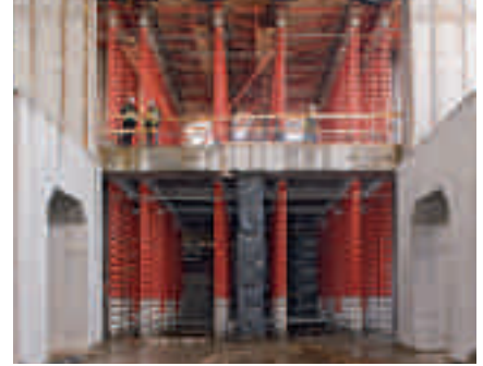
Transferring high loads with low space requirements – making full use of the advantages of the HD 200 Heavy-Duty Prop for the construction of a power plant.
