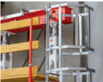
Ladders with safety cages, which are attached to the prop chords, guarantee safe access.
