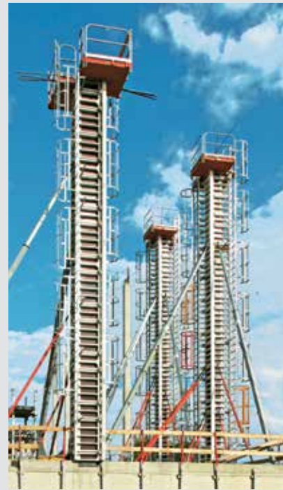
Concreting Platform, complete, Item-no.: 037400. Permissible load of 150 kg/m 2 .
